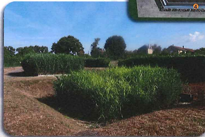
The reed bed sewage station
